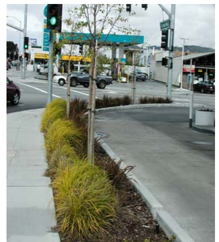
Figure 5.8 – Landscaping can provide a visual buffer between the roadway and adjacent pavement.
