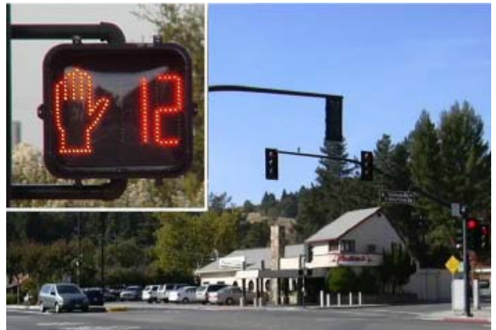
Figure 6.4 – Example of traffic signal mast arms and pedestrian countdown signals
