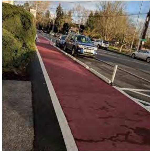
Sidewalk Extension; Seattle, WA; Photo: Dongho Chang
