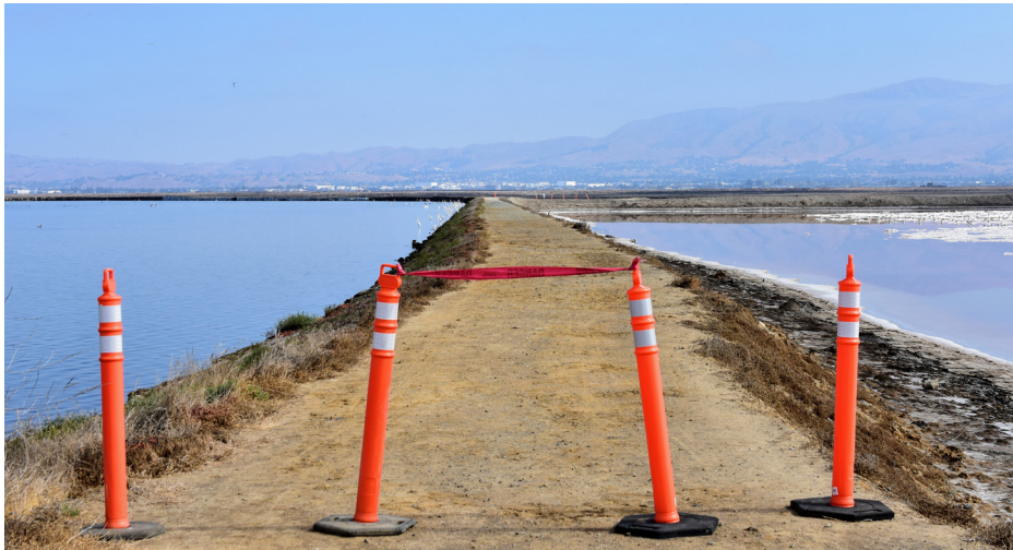
Alviso: Due to flood risks, temporary barriers prevent access to a segment of the Bay Trail. Photo Credit: ARUP
