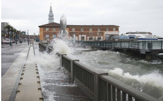
Photo: Port of San Francisco
