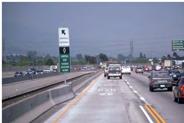
I-210 Pasadena, 1994 2-foot left shoulder, 11-foot lane, 1.5-foot buffer
