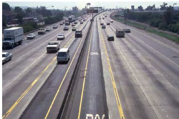
Initial operation by restriping shoulders
