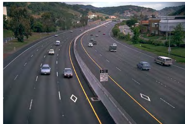
US 101, Marin County, 1990 4-foot left shoulder, 11-foot lane
