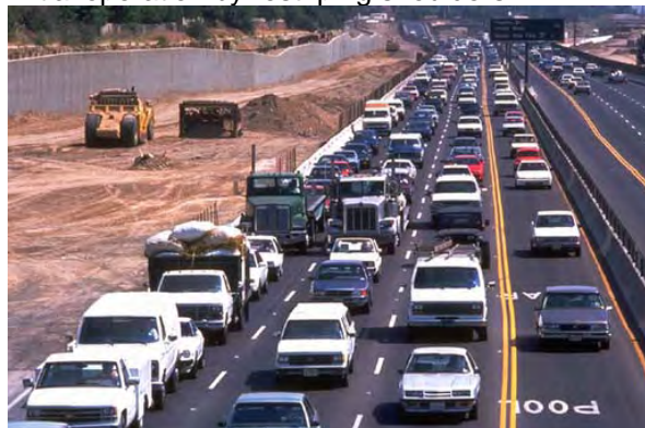
HOV operation during reconstruction
