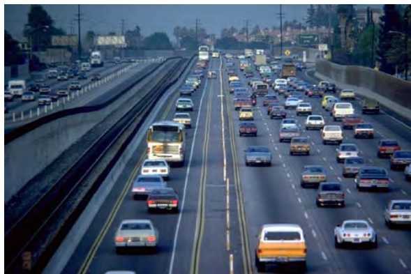
I-10 El Monte Busway, 1980 4-foot left shoulder, wide right buffer
