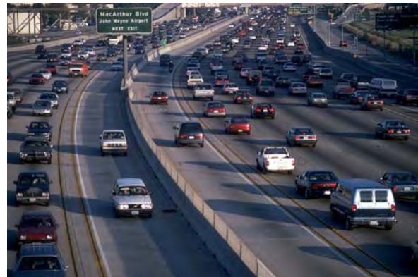
I-405, Orange County, 1995 4-foot left shoulder, 11-foot lanes
