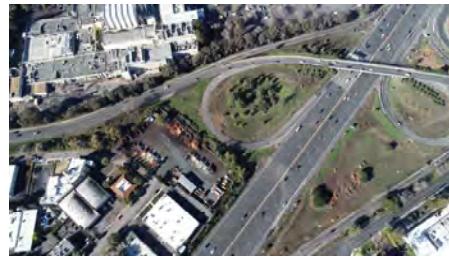
101/San Antonio Interchange – Lack of SB On-Ramp
