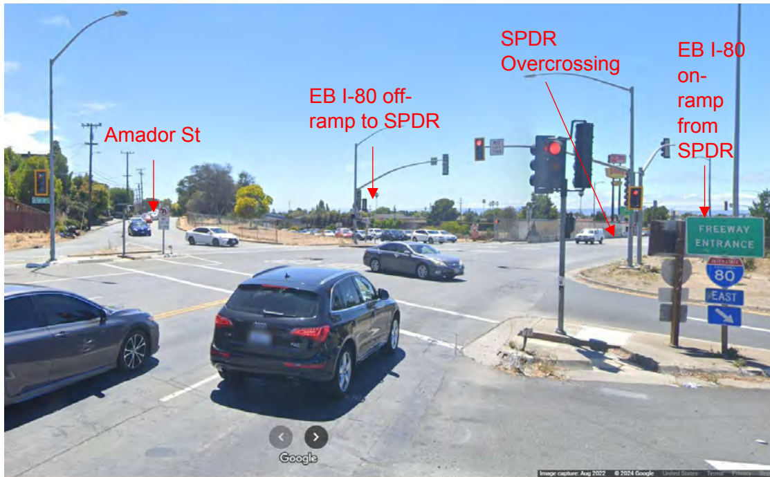
Figure 11. Top: aerial view. Bottom: view from westbound SPDR toward intersection with Amador Street (upper left of image) where no left turns are permitted due to close spacing of the SPDR eastbound off-ramp. Photo credit: Google. August 2022.
