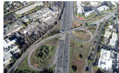
101/San Antonio Interchange
