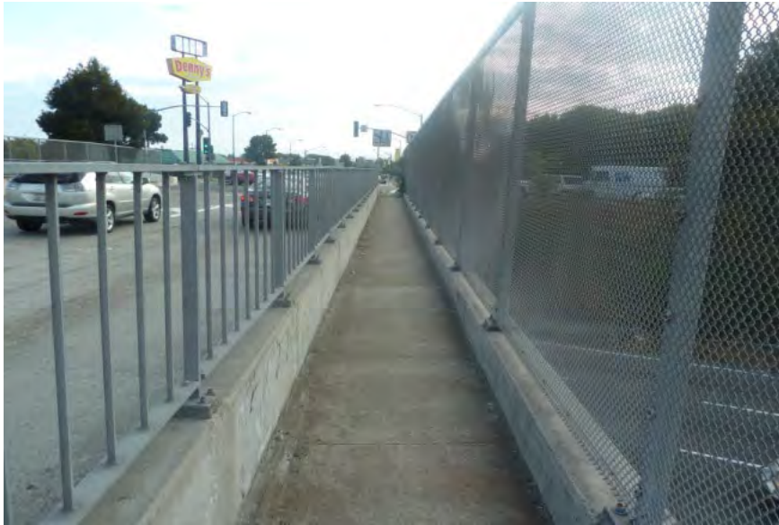
Figure 14. On SPDR overcrossing looking west, with 4-foot-wide sidewalk on north side of structure. Photo credit: AECOM.
