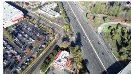
101/Rengstorff Interchange –SB On-Ramp Weave
