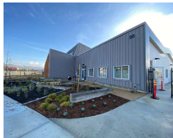
Photos of projects completed with RM 3 Capital Funding. Left – Mokelumne Trail Bicycle/Pedestrian Overcrossing of SR-4. Right – Vine Transit Maintenance Facility.
