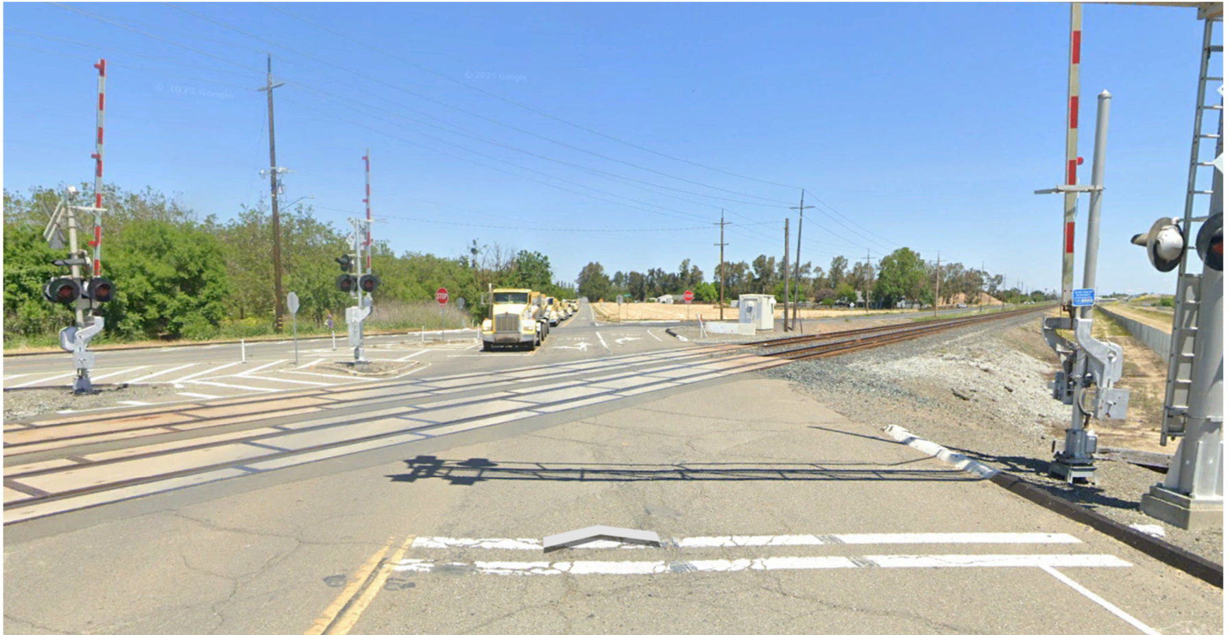
Figure 5: Pitt School Road/Porter Road Interchange – looking north on Pitt School Road
