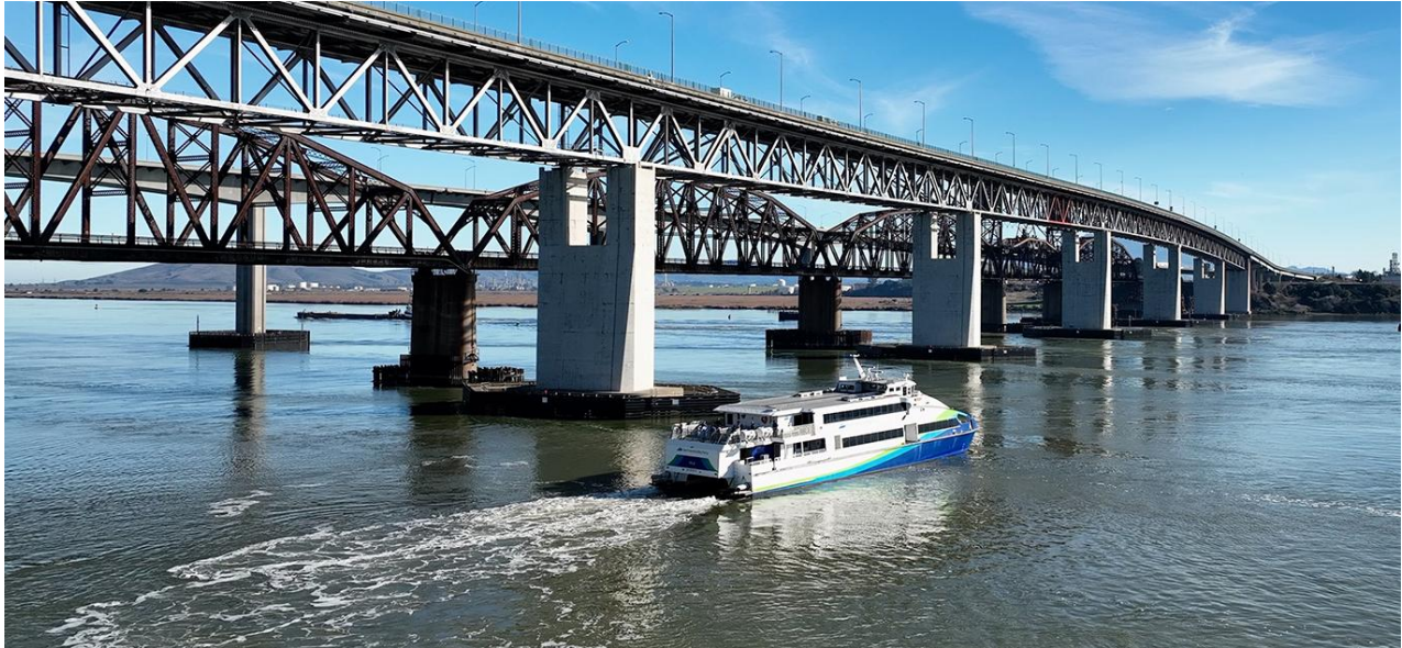
A WETA ferry carries state officials, BATA staff and others on an inspection tour of the Benicia-Martinez Bridge. Photo: Mark Jones, MTC
