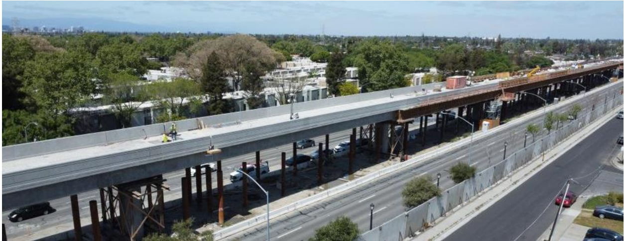
Aerial view of the superstructure under construction VTA images
