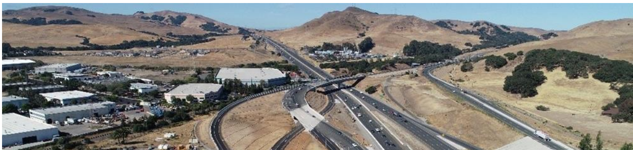
First RM3-funded construction package for the I-80/I-680/SR 12 interchange in Fairfield.
