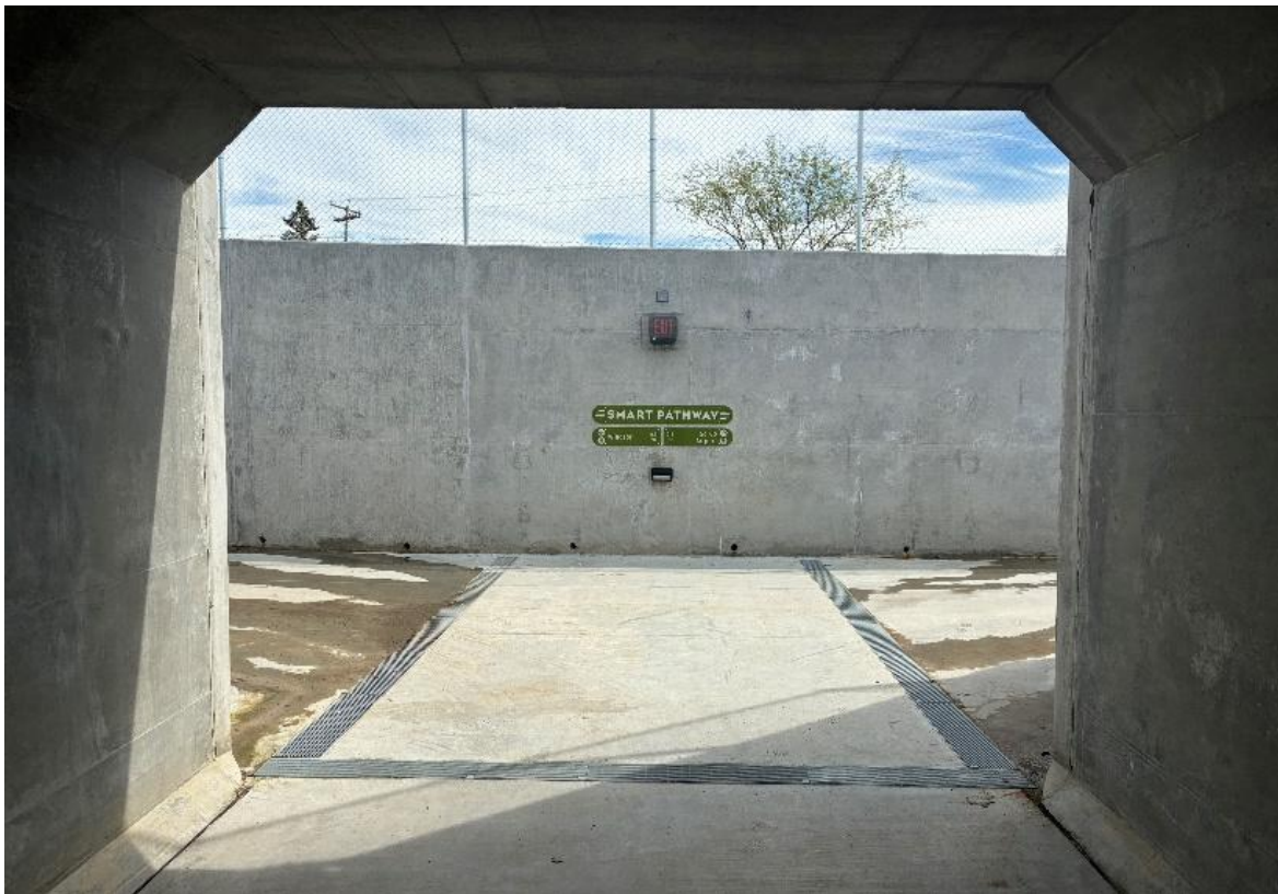
SMART Windsor High School Undercrossing. Photo: SMART
