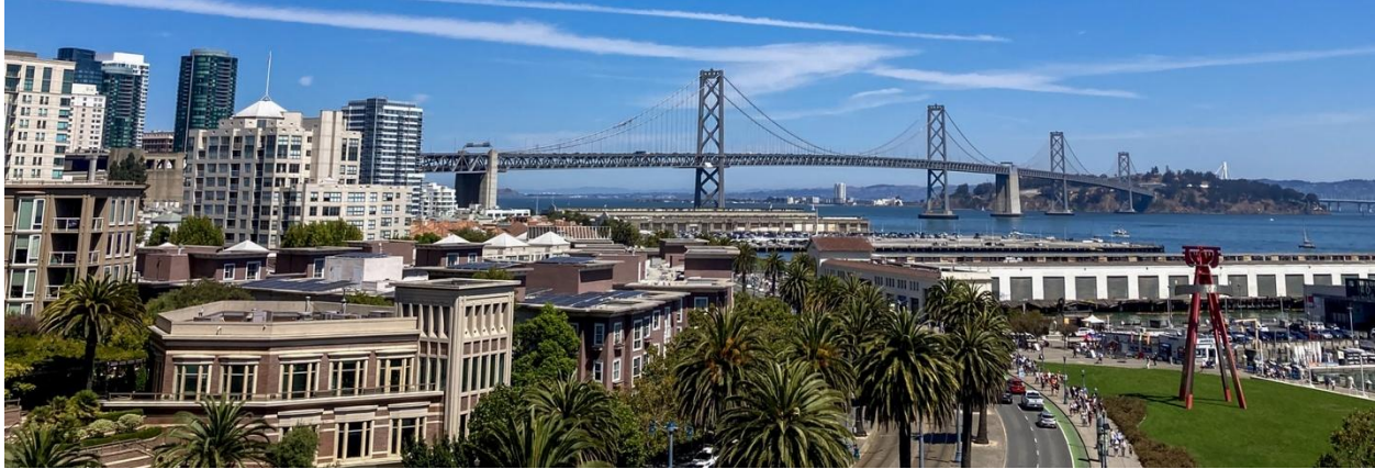
The West Span of the San Francisco-Oakland Bay Bridge on a beautiful day on the Bay. Photo: Joey Koffica, MTC.
