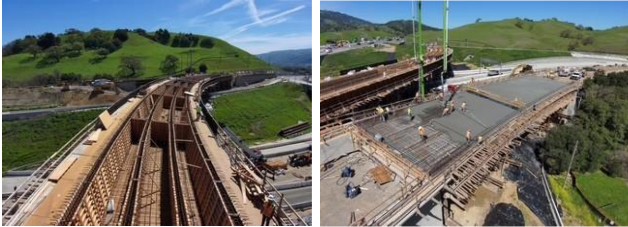
Construction progress on I-680/SR 84 Interchange Photos: Alameda County Transportation Commission
