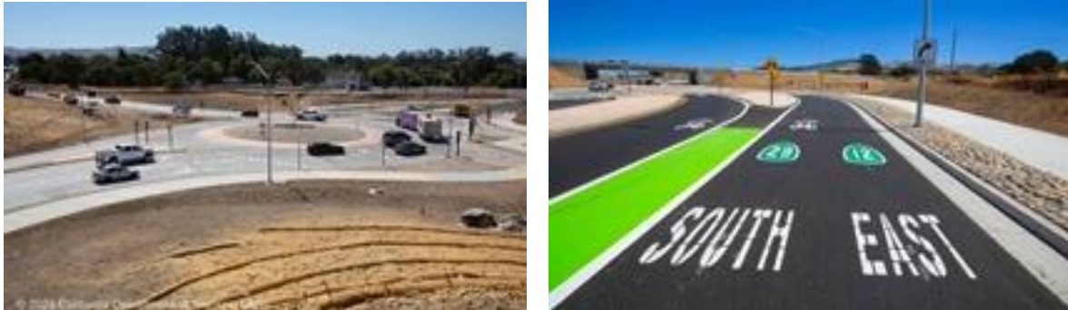
Left: Photo of Soscol Junction Roundabout. Right: Photo of Soscol Junction bike lanes. Photos: NVTA
