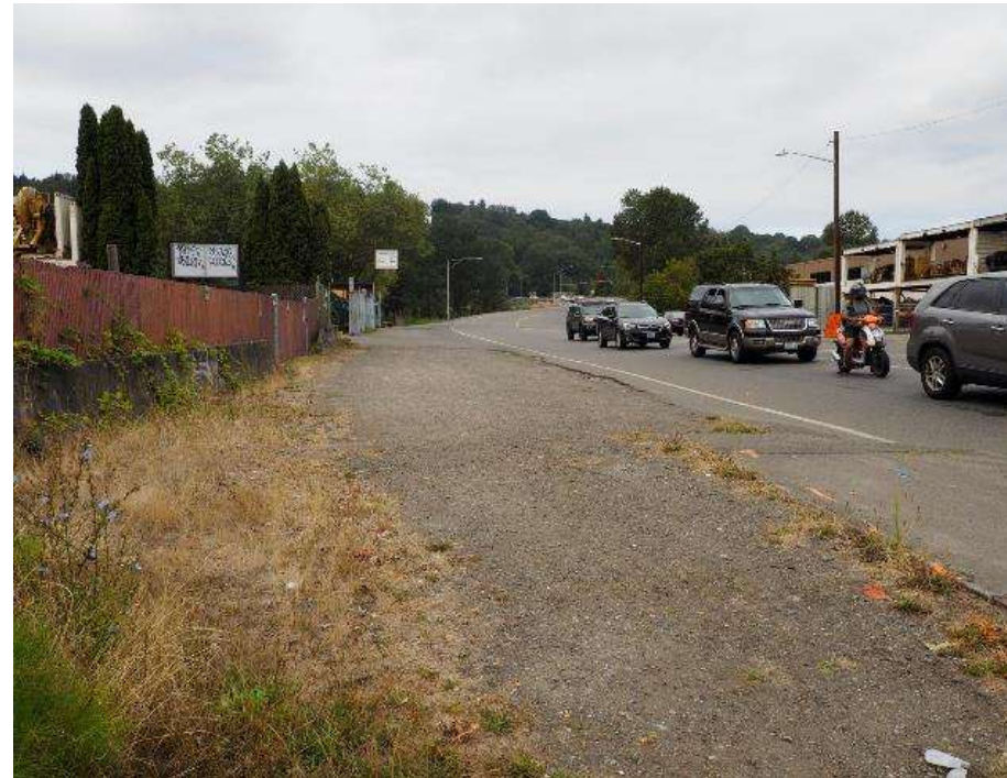
Example of street with an edge line and no sidewalk present. Source: Toole Design
