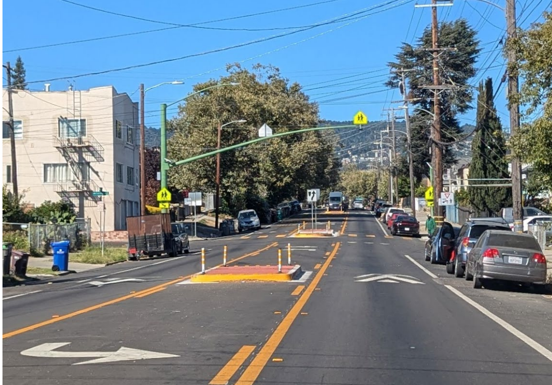
High Street Paving Project (Completed Spring 2024)
