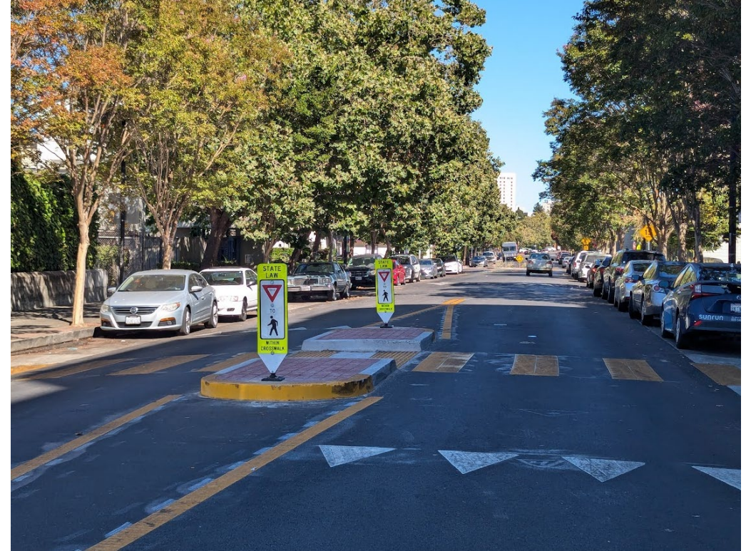
8 th Street West Oakland Traffic Calming Project (Completed Summer 2024)
