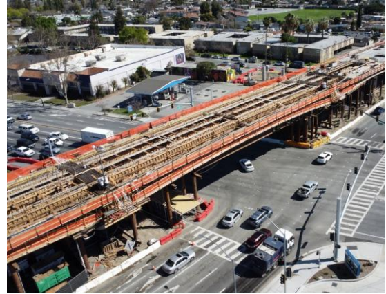
Right: Eastridge Regional Connector bridge construction at Story Road, VTA photo
