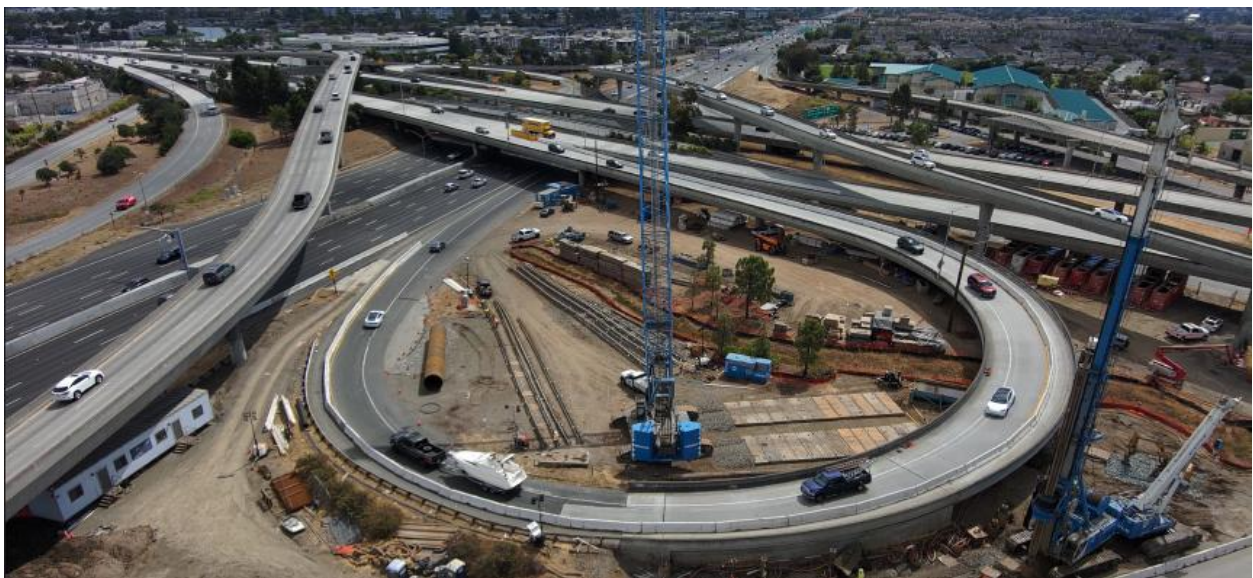
Top: US 101/SR 92 Construction Progress, SMCTA Photo
