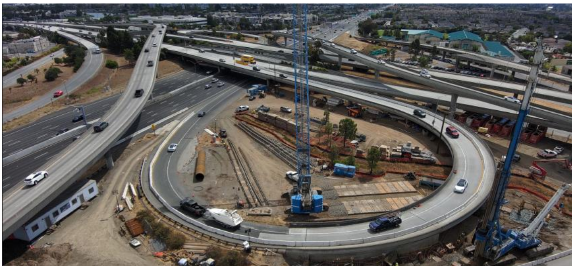
US 101/SR 92 Construction Progress SMCTA Photo
